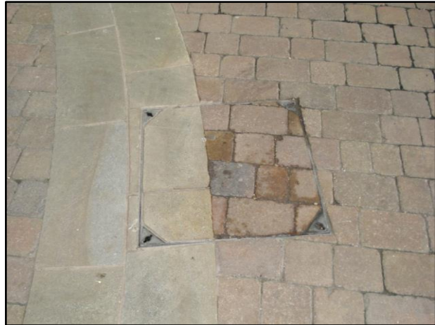
Acceptable high quality public realm utility reinstatement
