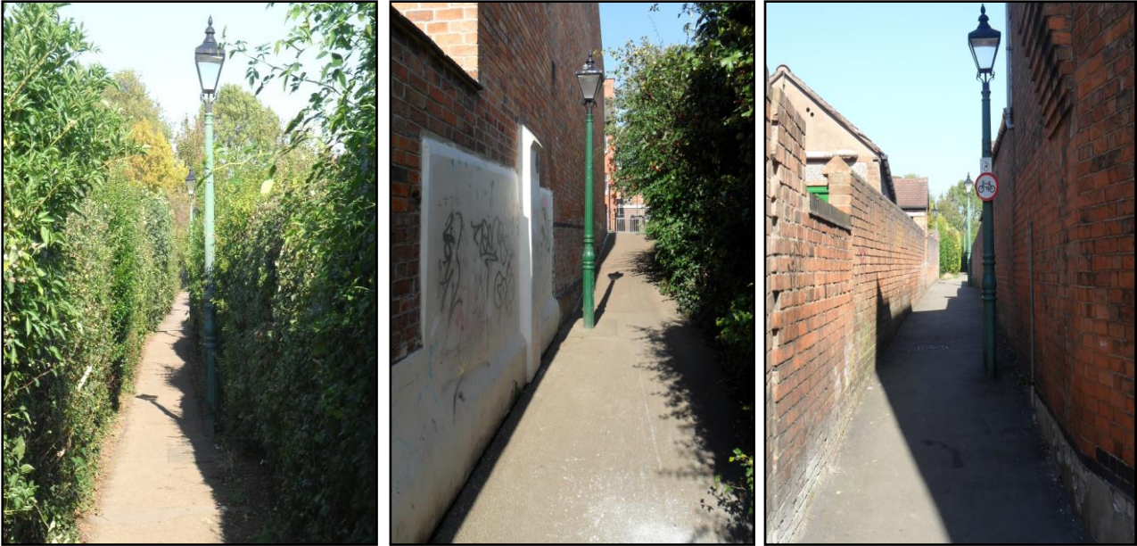
Illustrations of the condition of The Lanes in Wigston.
