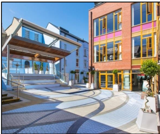
High quality surfacing materials, Derry.
