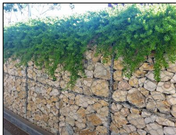
High quality example of planted stone gabions.
